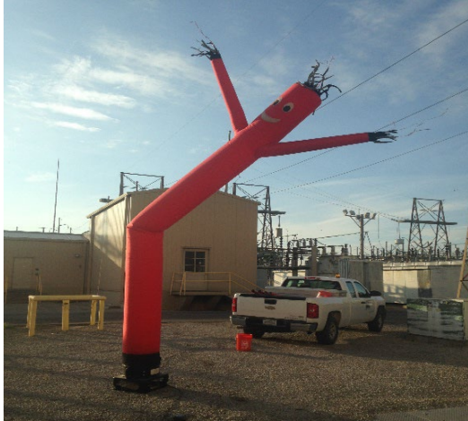
Figure 5. Air dancer installed at a facility to deter flocking birds.
