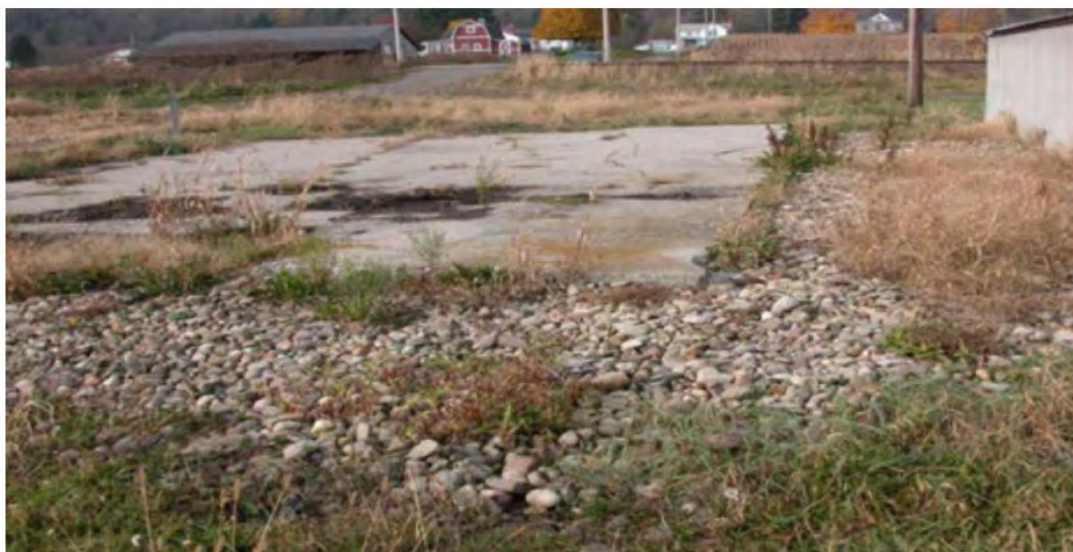
Figure 7-1 Sloped, Concrete Gravel Pad for Cleaning and Disinfecting Equipment
